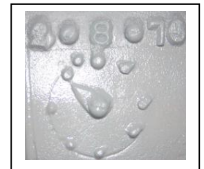
Reference 1970 340 engine casting date and manufacturing date wheel location on the RH side of the block
